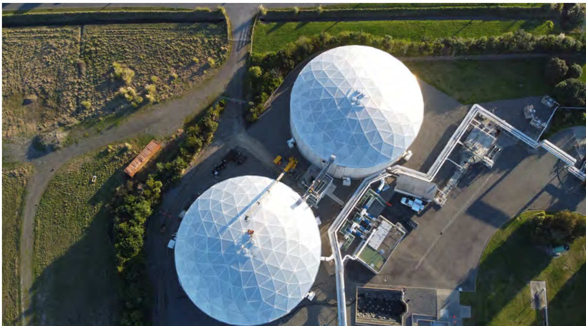
Figure 1: East Clive Wastewater Treatment Plant - Biological Trickling Filters
