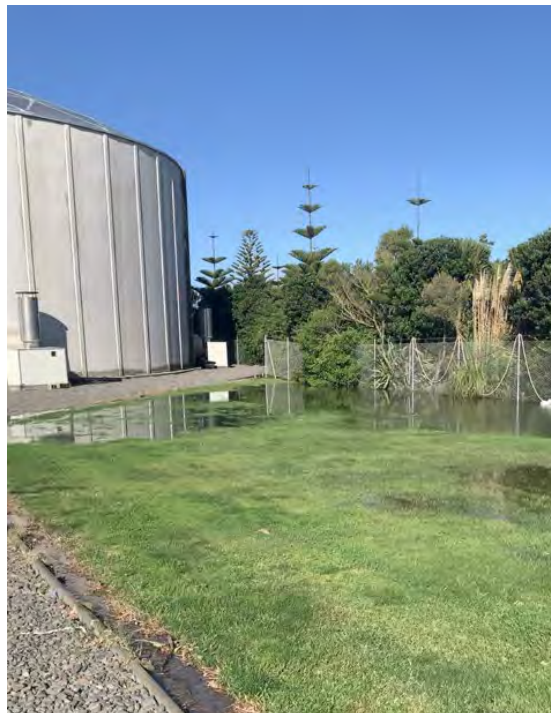
Figure 6: Wastewater spill overland flow towards Grey Street roadside drain
