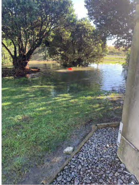
Figure 5: Domestic wastewater Inlet manhole (East Clive WWTP spill location)
