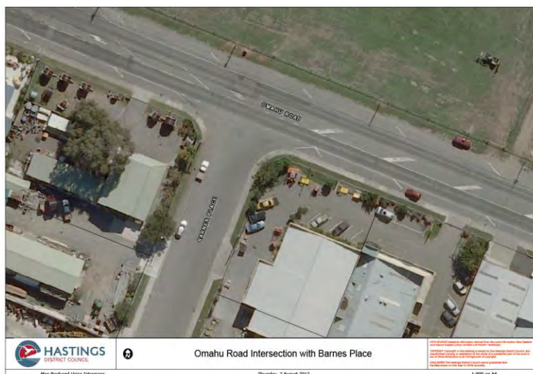
Figure 8 (Barnes Place Intersection- Pre Road Renewal)
