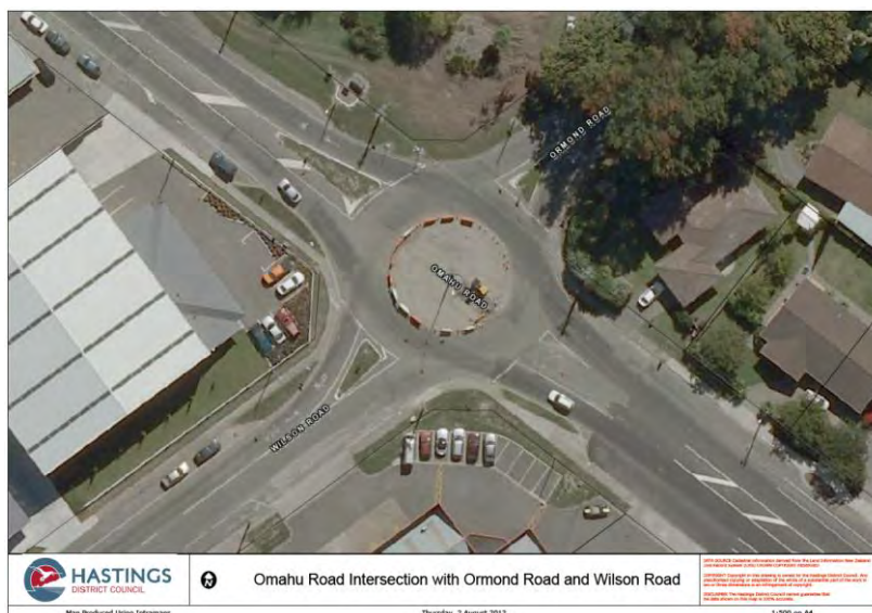
Figure 12: Ormond Road/Wilson Road Intersection - Pre Road Renewal
