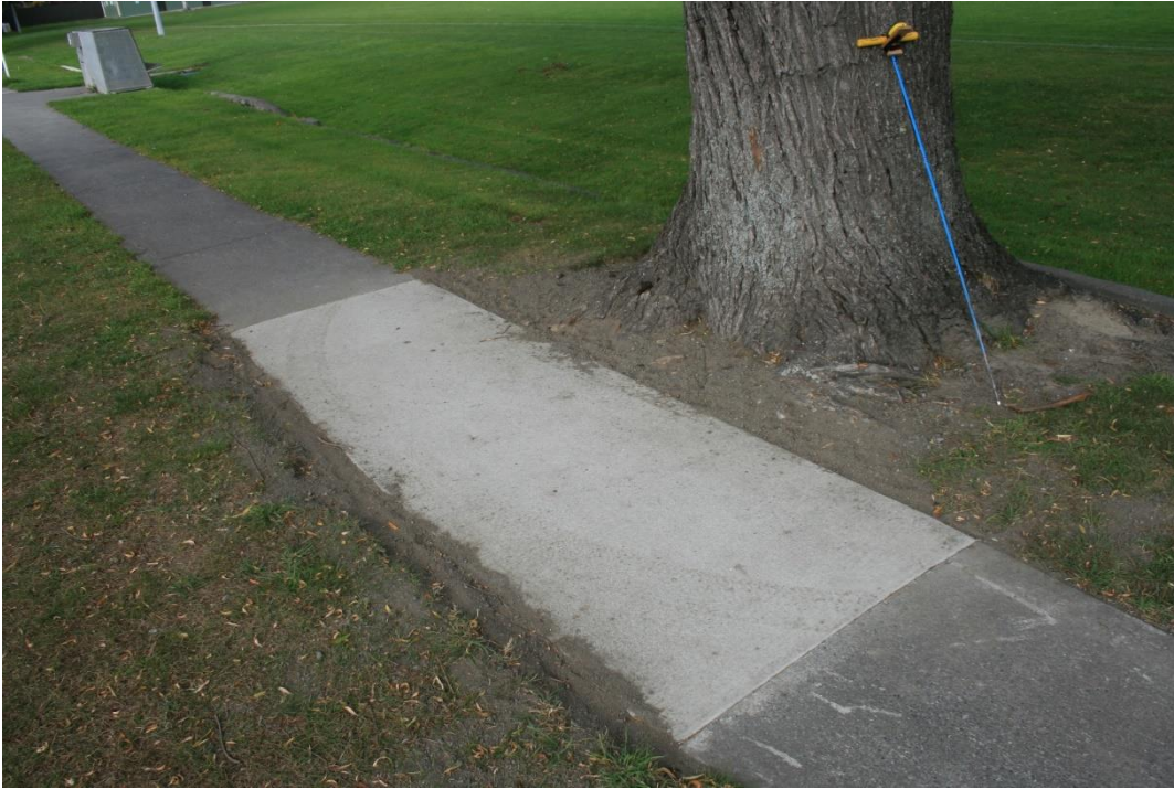
Fig.19 New section of pavement within root zone of willow
