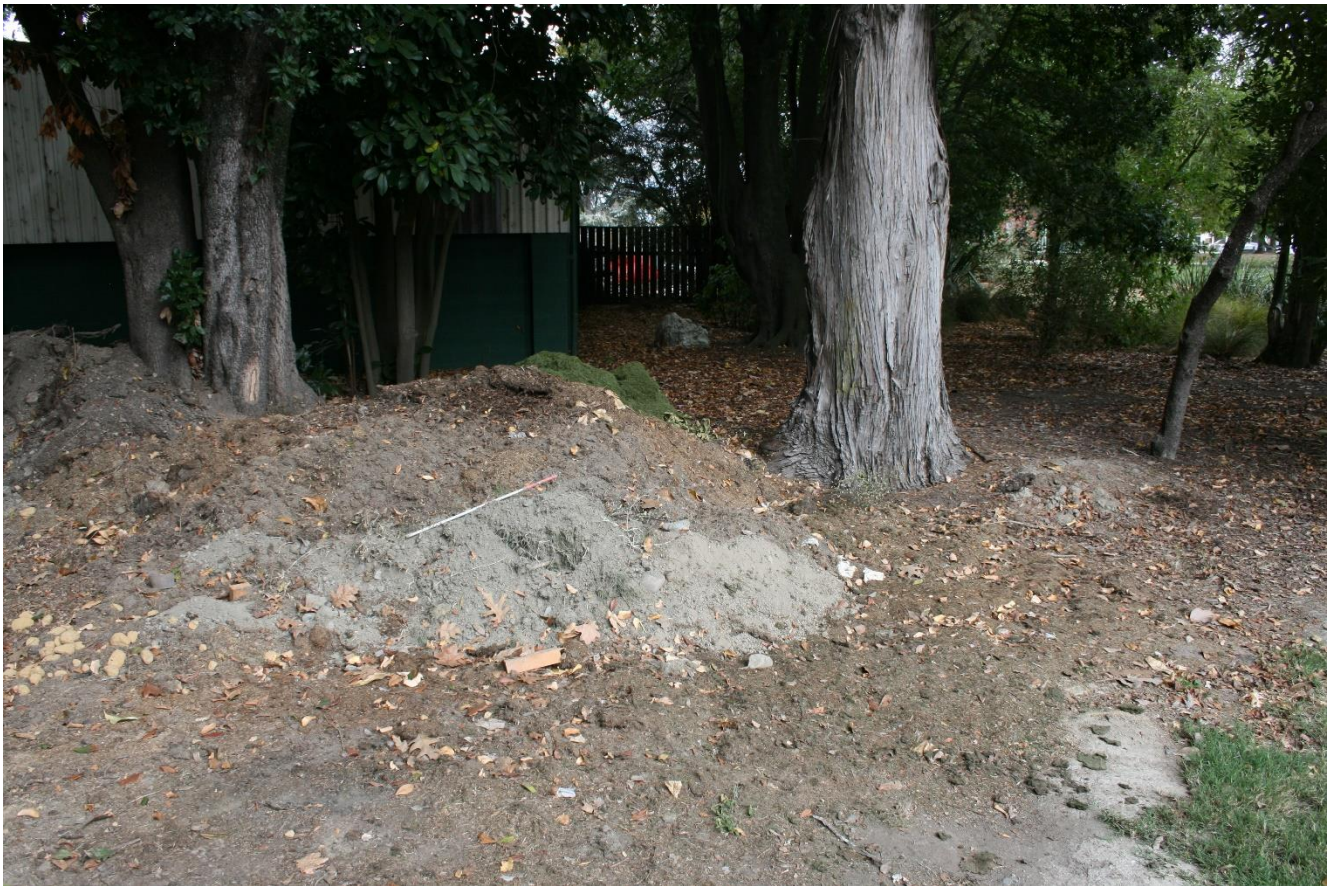
Fig.21 Close up of the damage. The extensive build-up, damage and debarking of a rare Picconia excelsa (left of image) by depot.
