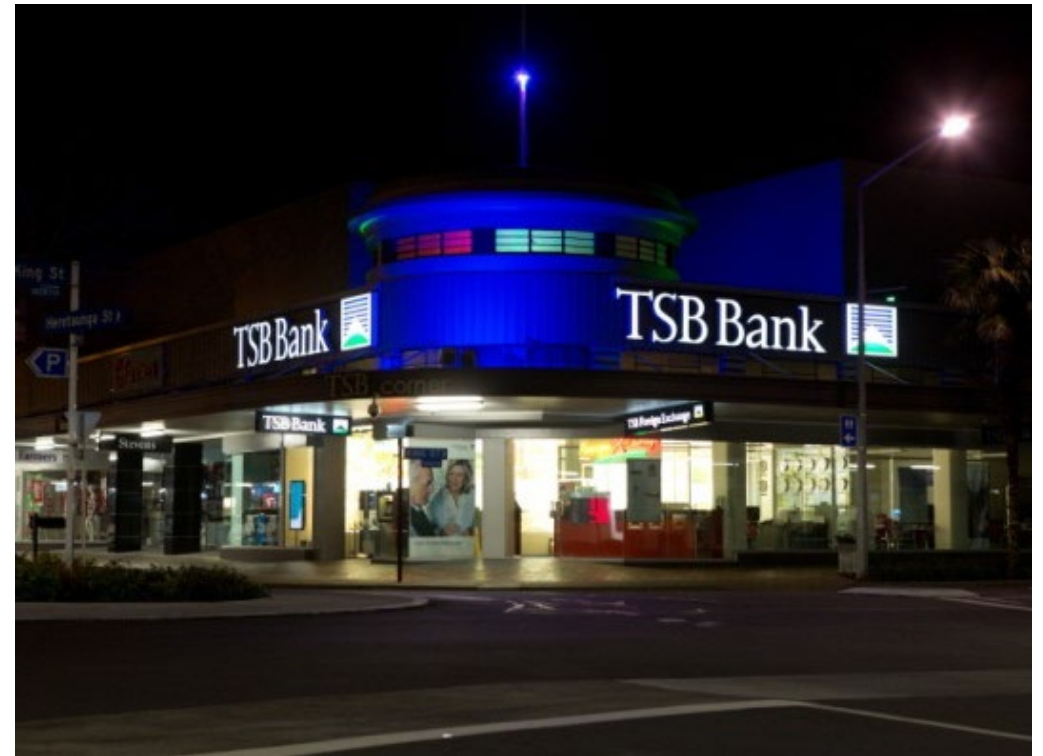
Heretaunga Street West
