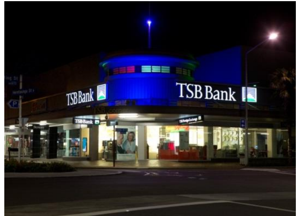
Heretaunga Street West
