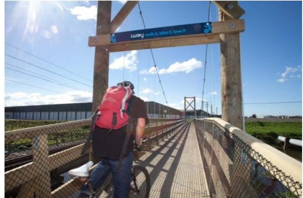
A completed part of the iWay Walking and Cycling network.
