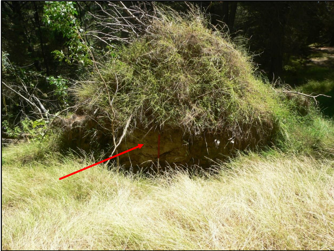
Figure 10 Example of damage occurring to pā and potential associated public safety risks through uncontrolled tree fall: scale (arrowed) = 1 m.
