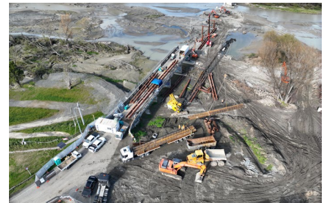
Waiohiki/Redclyffe Bridge. Photo: WSP
