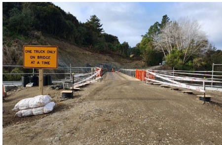
Mangatutu Bridge, Photo: Fulton Hogan
