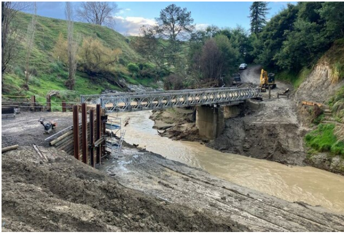
Moeangiangi bailey bridge
