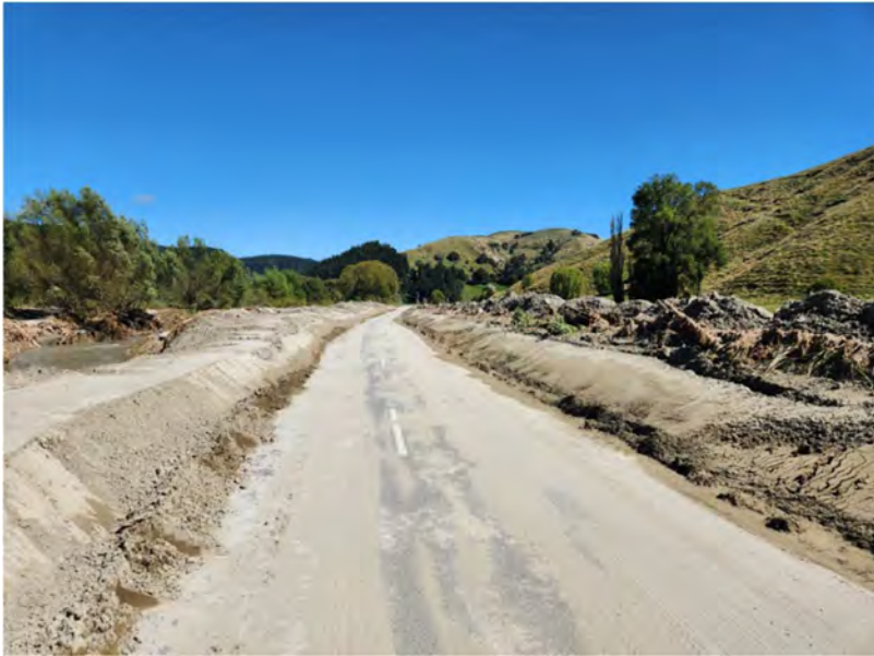
Figure 2.7: Silt buildup excavated from Beach Road orientated west, Source David Colville
