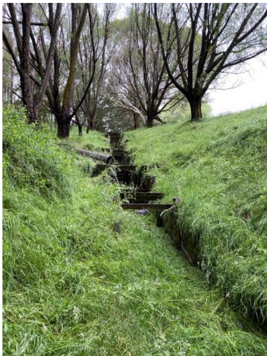
Figure 17: Spillway looking upstream (very long vegetation)
