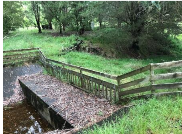
Figure 14: Livestock gate across spillway
