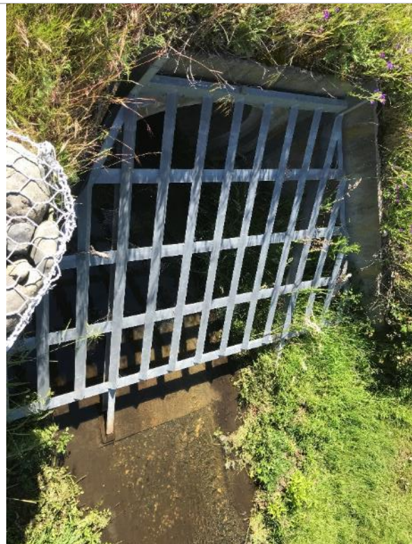
Figure 58: Screen at intake structure
