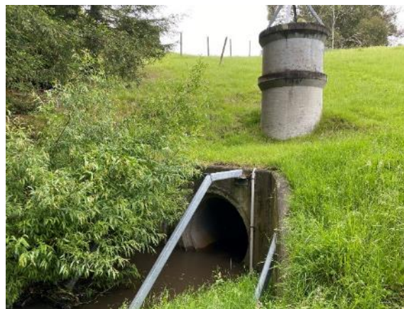
Figure 42: Inlet structure (bush to be removed)
