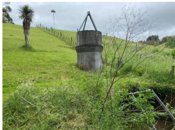
Figure 33: Auxiliary intake and inlet structure (blocked with log)
