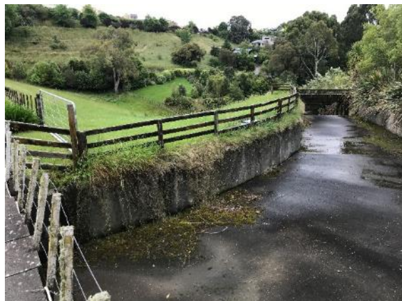
Figure 28: Narrowing of upper spillway channel
