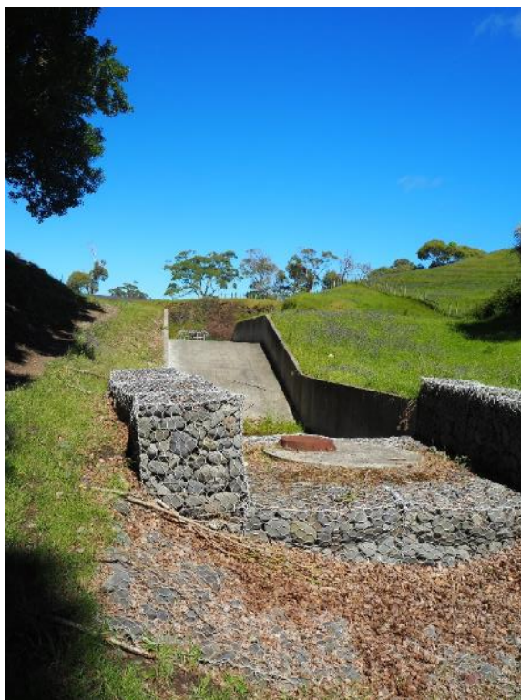
Figure 57: Downstream slope and spillway
