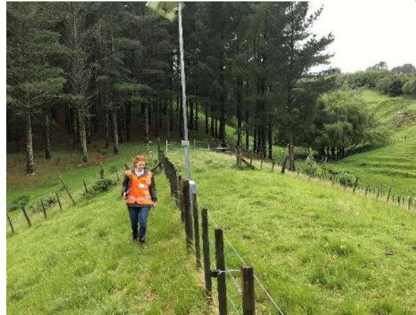
Figure 2: Dam crest with weak fence
