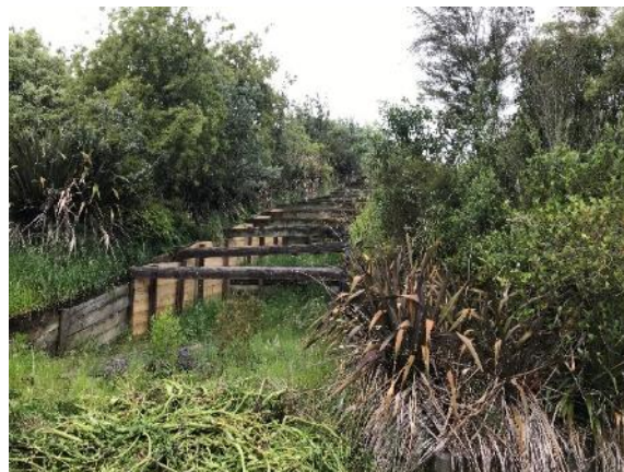
Figure 29: Timber spillway channel looking upstream (repair is lighter wood)
