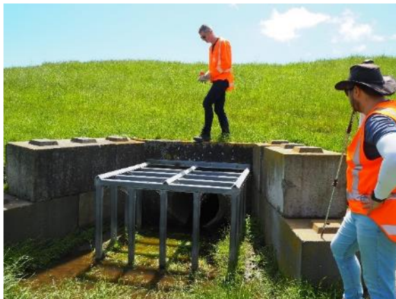
Figure 49: Inlet structure on central dam, noting slight settlement in the vicinity of the pipe.
