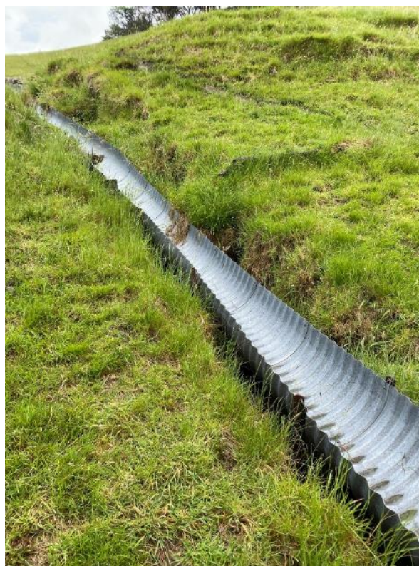
Figure 6: Spillway (low flow channel at end of spillway)
