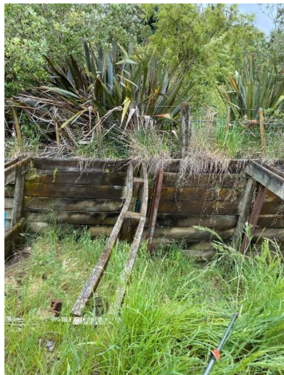
Figure 27: Buckling cross timbers in spillway
