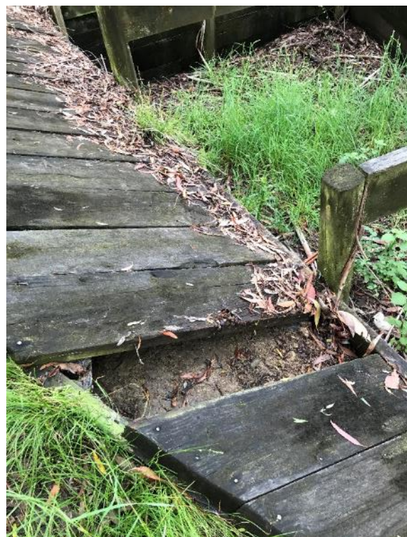
Figure 16: Missing timber on spillway
