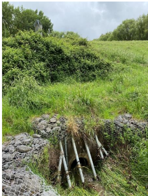
Figure 12: Screened inlet headwall structure
