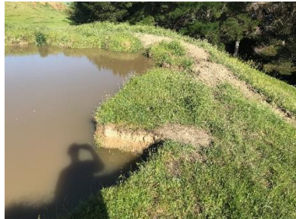
Figure 62: Downstream edge of failing pond (for cattle drinking water) above Western Dam
