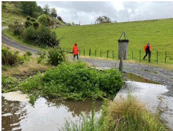
Figure 24: Inlet structure (blocked, subsequently cleared)
