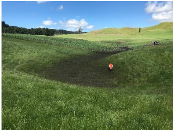
Figure 51: Evidence of recent ponding at east dam inlet pipe
