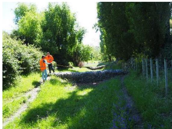
Figure 60: Spillway and gabion check dams
