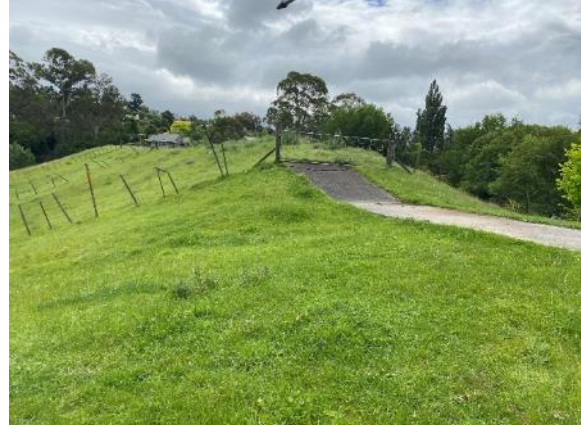
Figure 37: Spillway sill and 'natural' dam crest / right abutment
