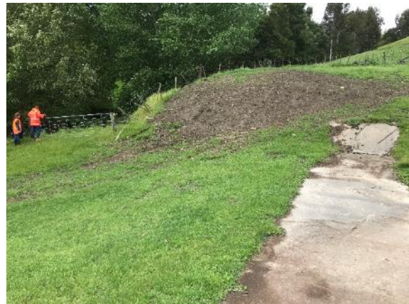
Figure 35: Spillway and recent repair to right hand side
