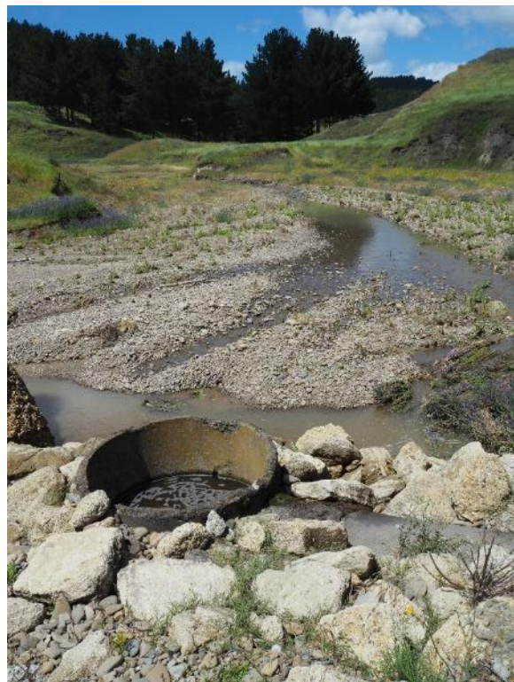
Figure 54: Outlet to Charlton Stream. Screen Required,
