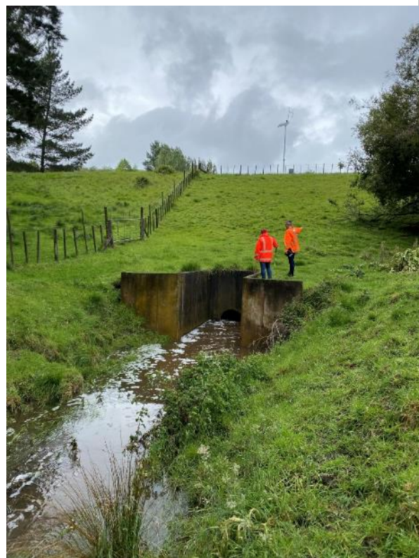
Figure 4: Outlet headwall and downstream face
