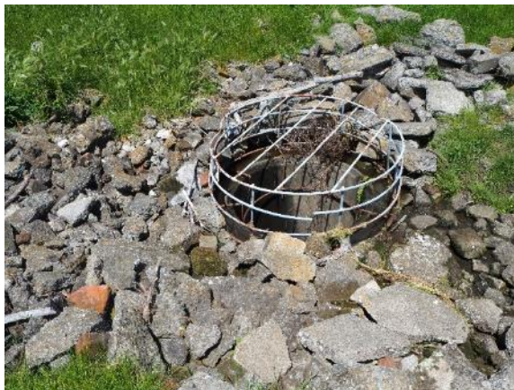
Figure 53: Downstream drop structure to Charlton Stream
