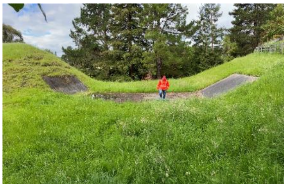
Figure 45: Spillway control sill
