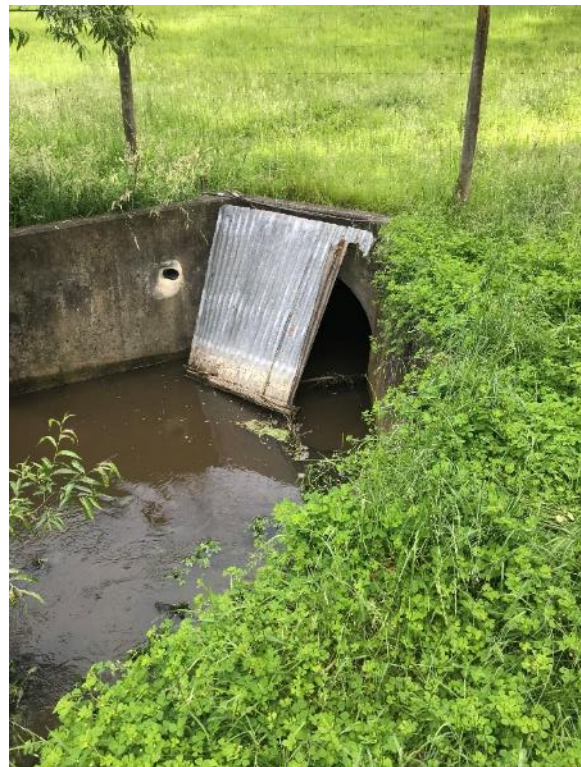
Figure 44: Culvert outlet with flap gate
