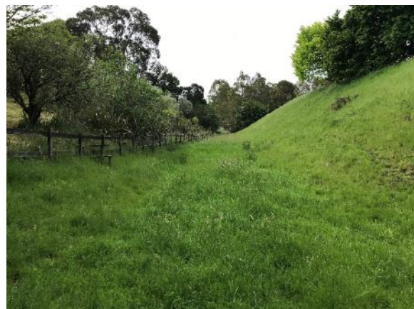
Figure 46: Spillway (undesirable fence / vegetation on the left-hand side and closed gate at the end of the channel)
