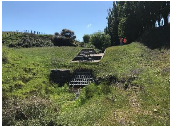
Figure 56: Upstream slope, spillway, and intake structure with auxiliary intake
