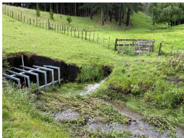
Figure 3: Screened inlet headwall with side inlet
