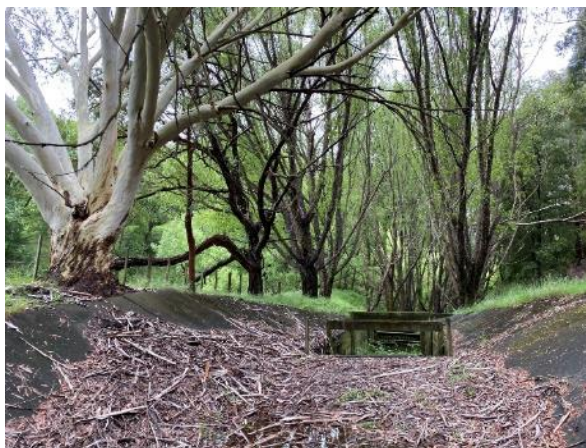
Figure 15: Spillway (showing tree roots probably lifting slab)
