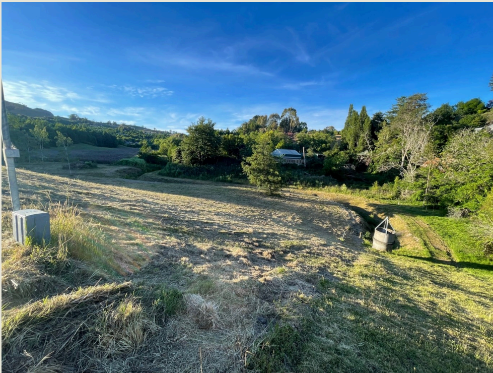
Figure 1: Mangarau dam mowing and fence readjustment.
