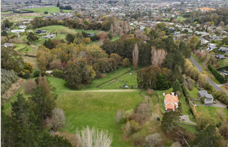
Figure 4: Herehere Dam looking down into Havelock North, dam crest (wall) in middle of photo and stream channel running down middle of photo
