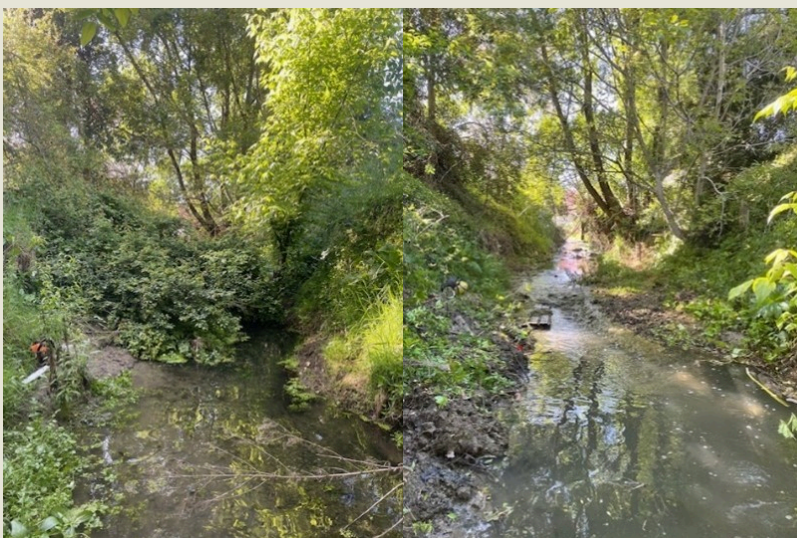
Mangarau Stream debris clean up
