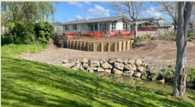
Mangarau Stream repair works to Drainage/ stream Embankment
