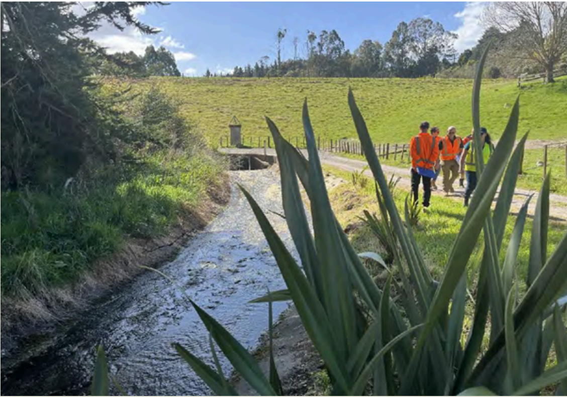
Engineers inspecting the Te Kahika Dam
