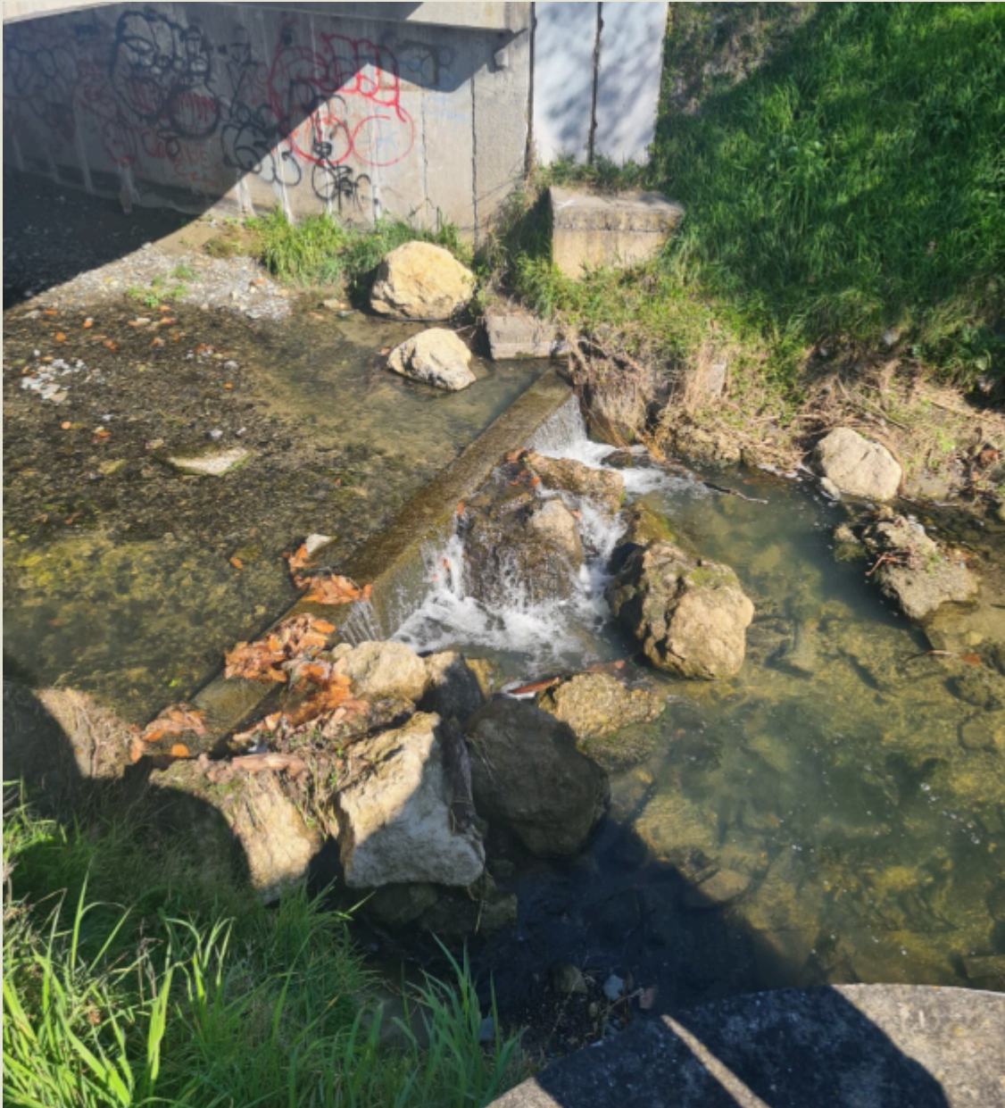
A concrete grade control structure on the Herehere Stream
