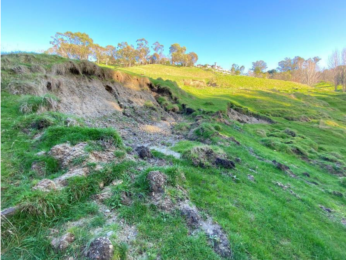
Figure 9-10. Landslides along the valley slopes (downstream of Spillway Downstream Structure).
