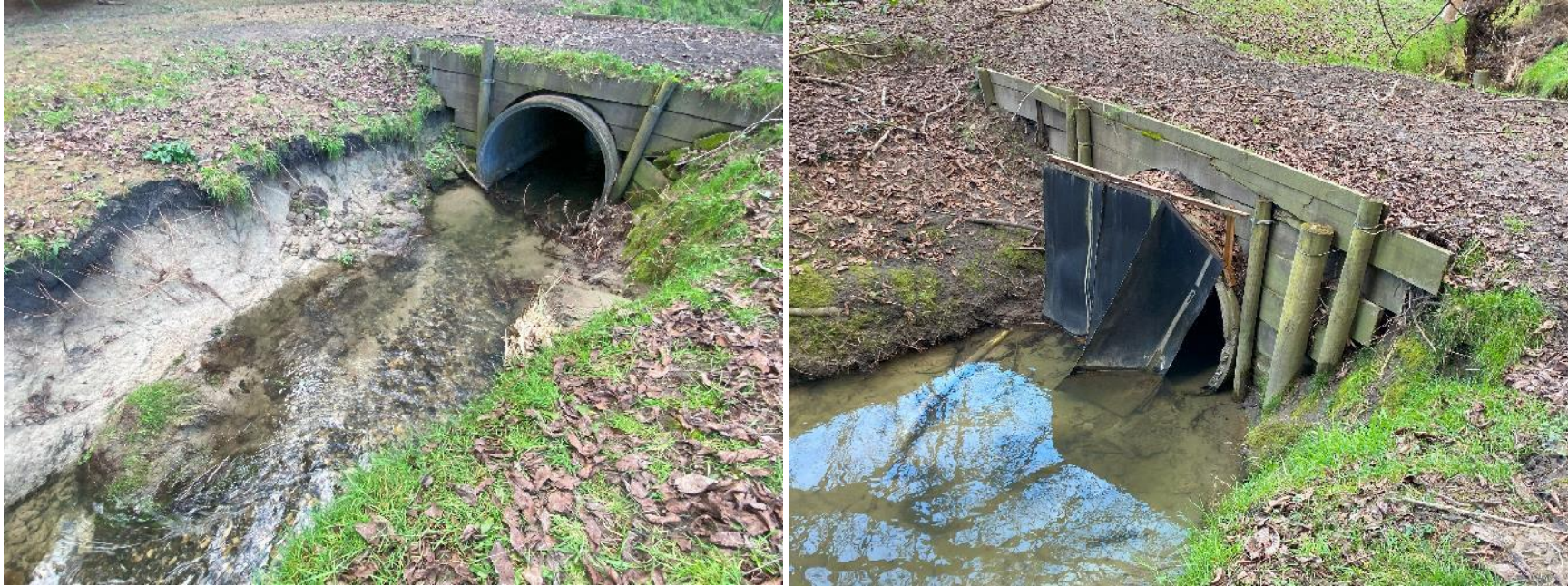
Figure 9-20. Upstream Channel Culvert for access track
