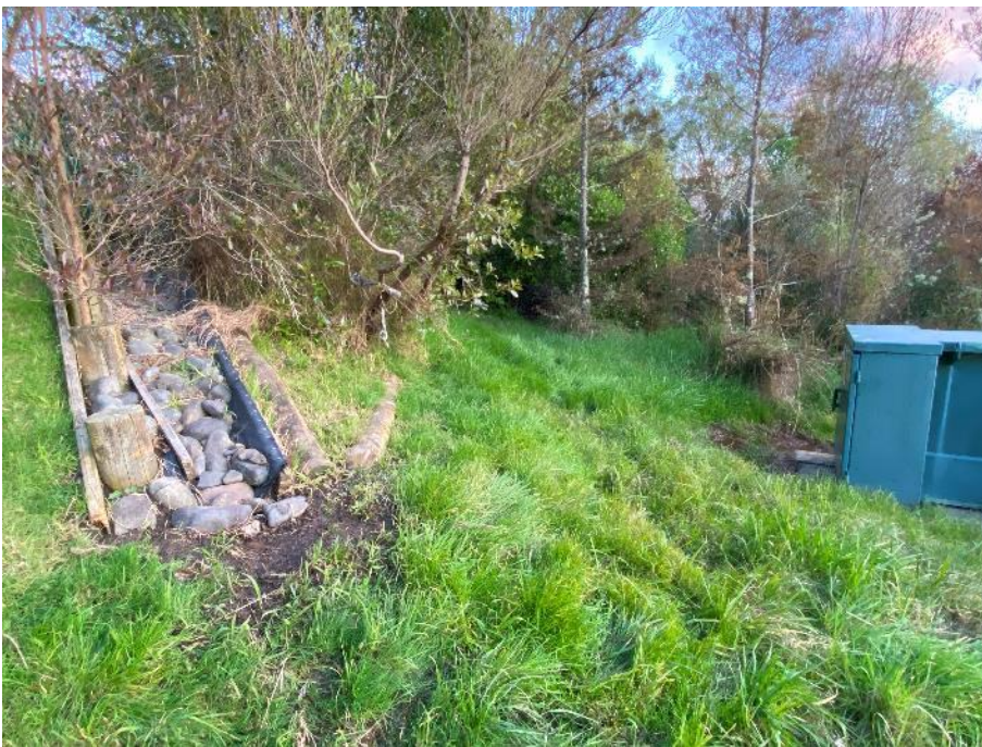
Figure 9-15. Wet patch on Downstream Right Abutment.
