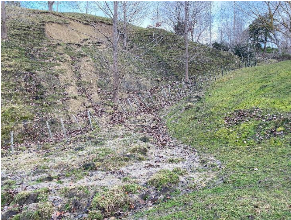
Figure 9-12. Landslide on Upstream Left Abutment.
