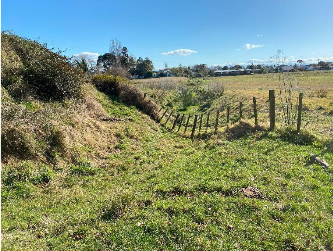
Figure 9-6. Lower: Spillway downstream channel below gabion walls.
