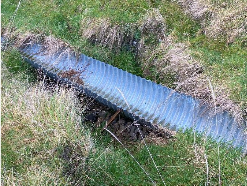
Figure 9-9. Spillway Downstream Structure
