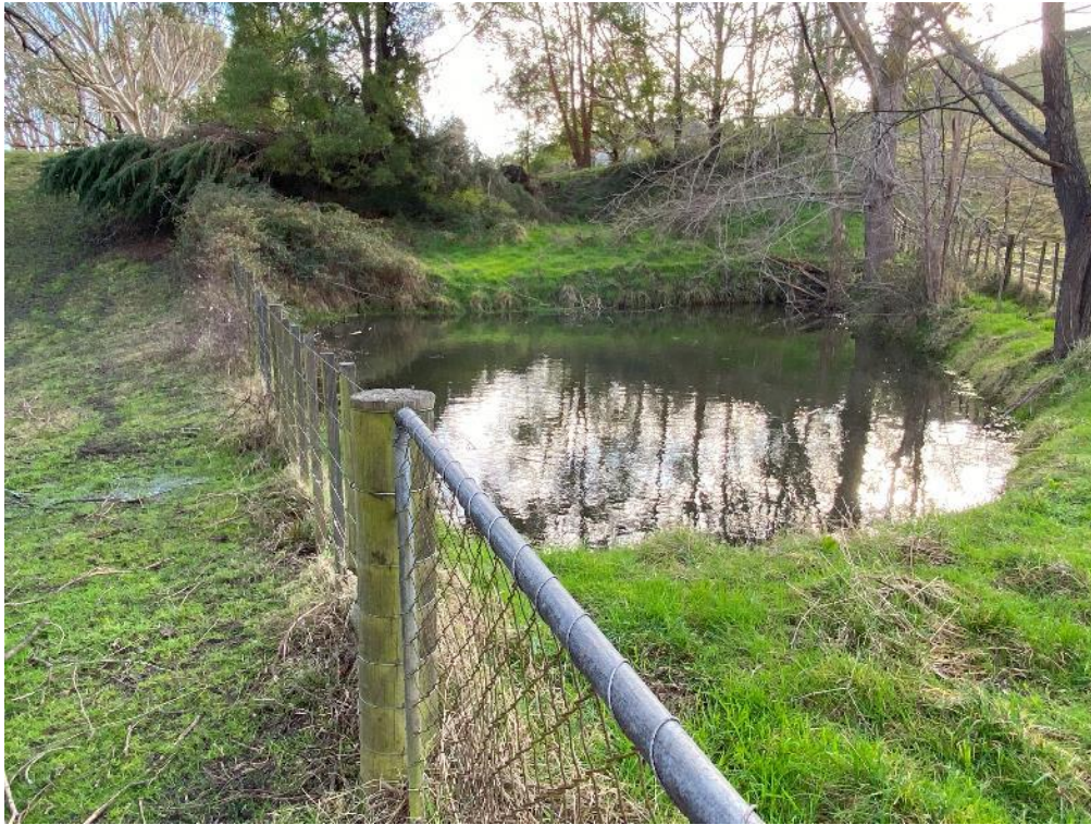
Figure 9-13. Pond in front of Right Abutment and Spillway.
