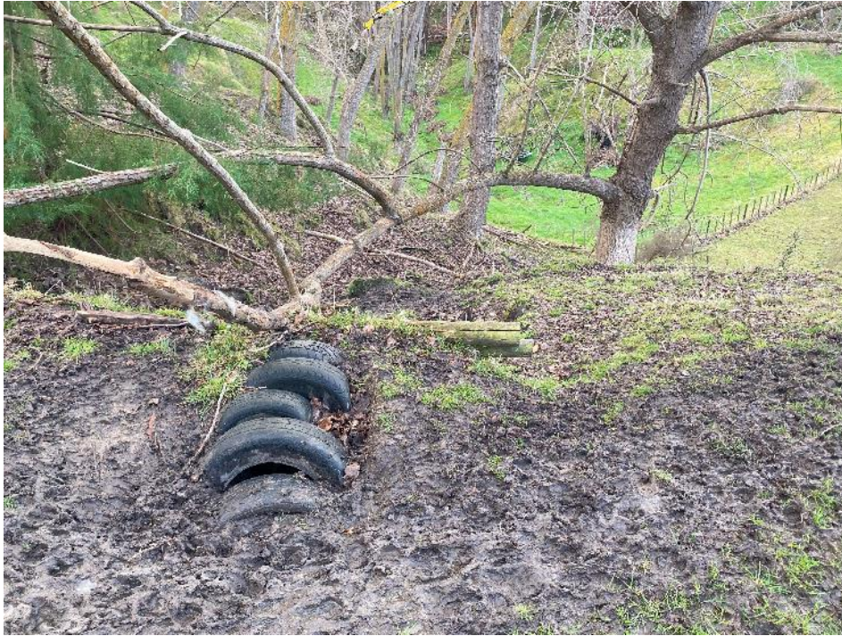
Figure 9-11. Drains under access path.
