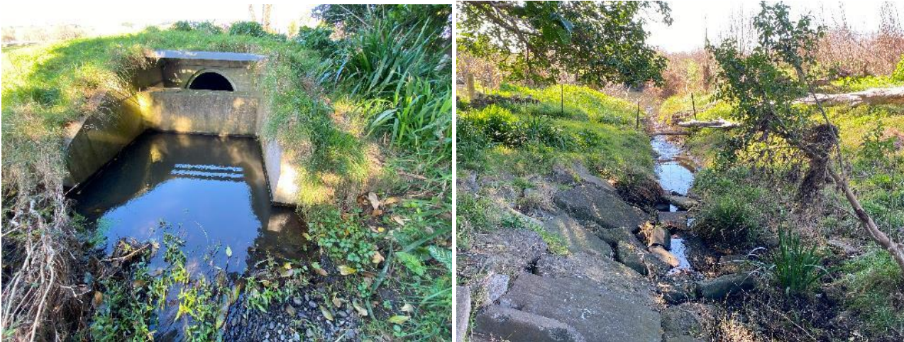
Figure 9-5. Lower: Outlet structure and channel to Maraetotara River.
