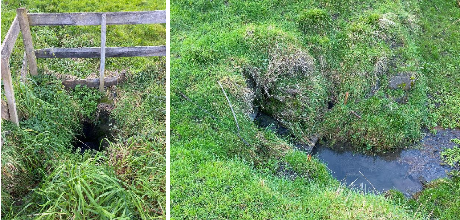
Figure 9-8. Side Channel (RHS of inlet) culvert inlet and outlet.
