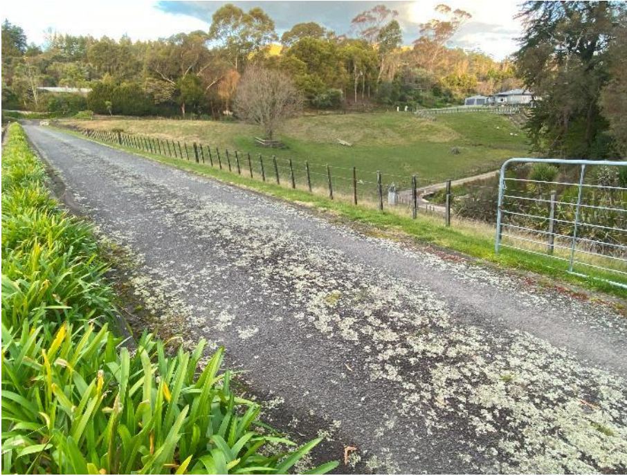
Figure 9-14. Dam Crest driveway.
