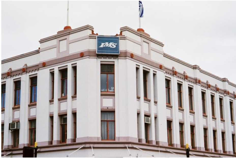
Close up of façade (R. O'Brien, NZHPT, 24 March 2006)
