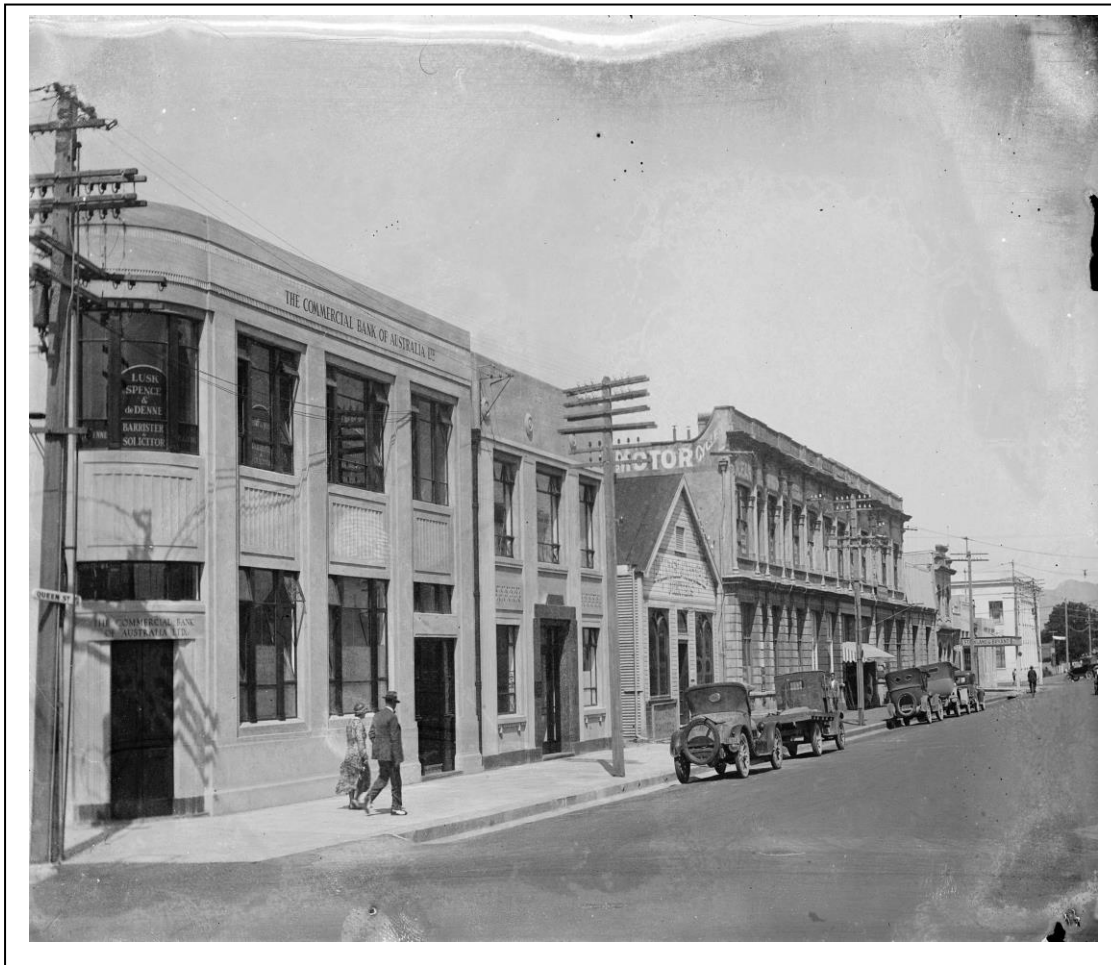
Commercial Bank of Australia Building (left) circa 1932 (Hastings, Streets, Queen, ca 1932, Henry Norford Whitehead, G-49405-1/2, Alexander Turnbull Library)
