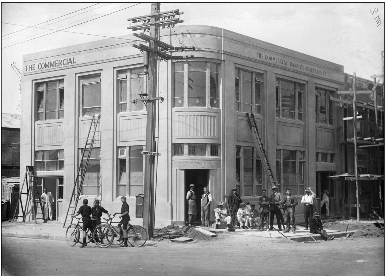
Commercial Bank of Australia Building (left) circa 1932 (Hastings, Banks, Commercial Bank of Australia Ltd, Henry Norford Whitehead, G-49408-1/2, Alexander Turnbull Library)
