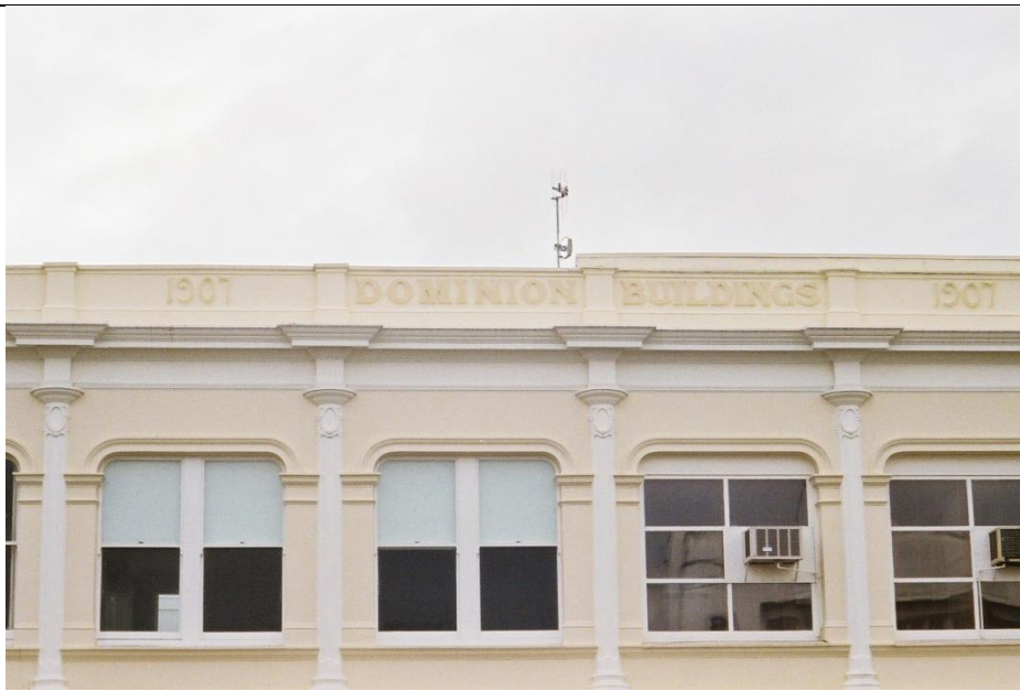
Details of upper level of façade (R. O'Brien, NZHPT, 24 March 2006)
