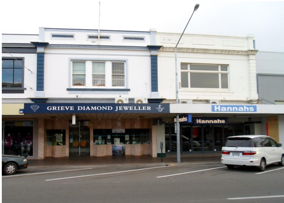
Building 3, 236 Heretaunga Street West, and Building 4, 240 Heretaunga Street West, 2012 (Building 3 on the left) (Photo: R. Murray)
