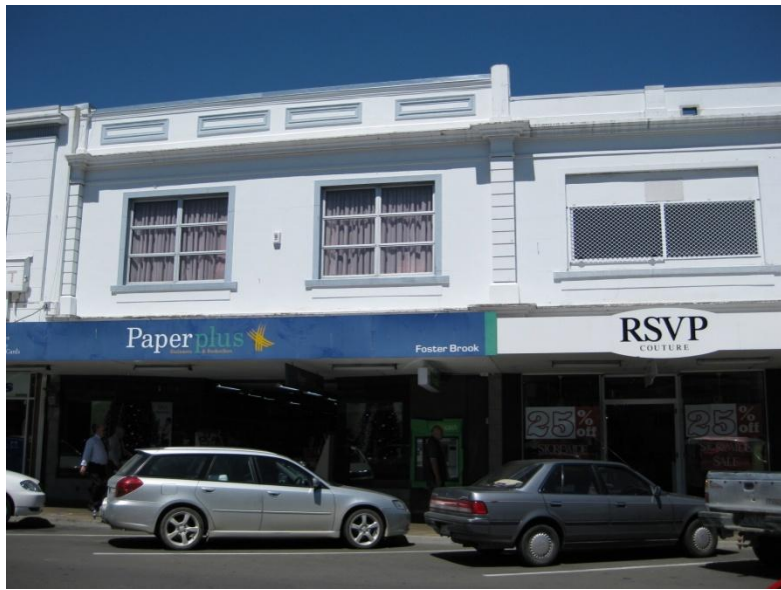
Building 1 and 2, Commercial Group #2 (S. Akers, 2009).
