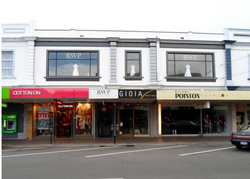
Building 2, 232 Heretaunga Street West, 2012 (Photo: R. Murray)
