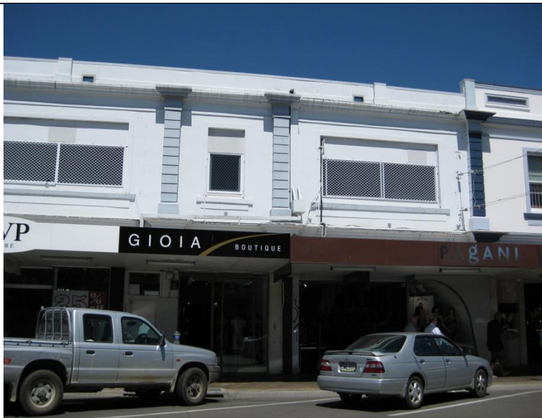
Building 2, Commercial Group #2 (S. Akers, 2009).
