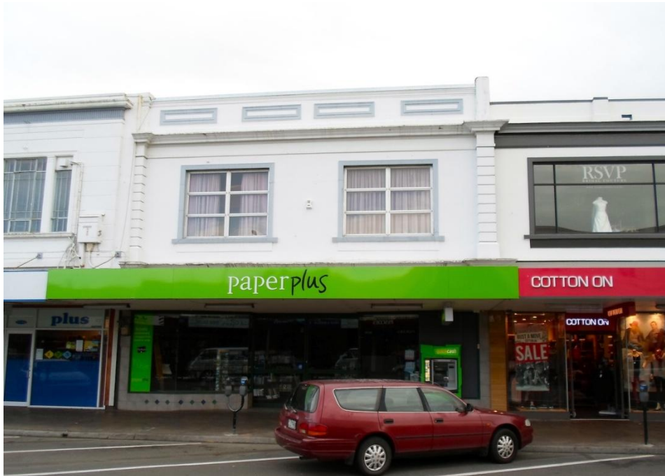
Building 1, 226 Heretaunga Street West, 2012 (Photo: R. Murray)
