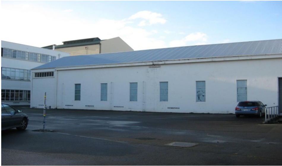
Municipal Power House, West Elevation, K Pascall, July 2012
