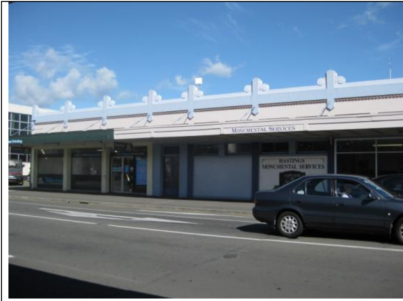
Nelson Street South view of King's Buildings (Sarah Akers, 2009).
