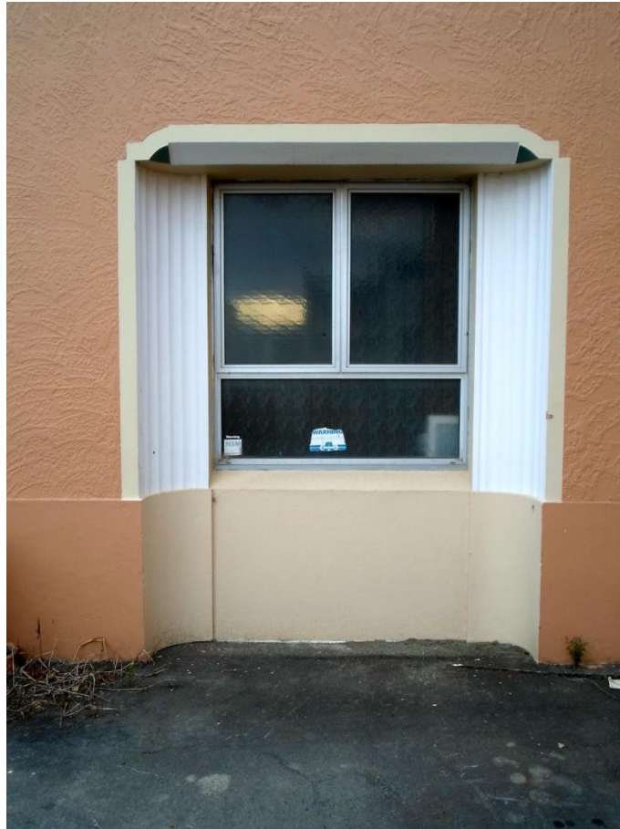
Modified door opening (infilled for window), 2012
