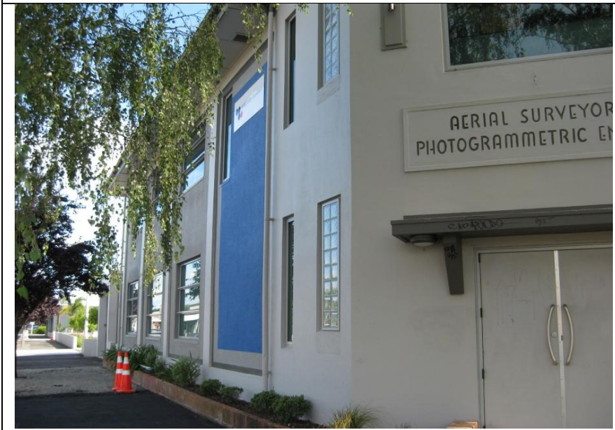
Avenue Road East façade of National Mapping Centre (S. Akers, 2009).
