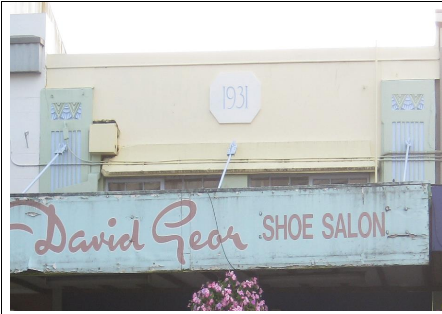
Close up of Building 1 façade (Sarah Akers, 2009)
