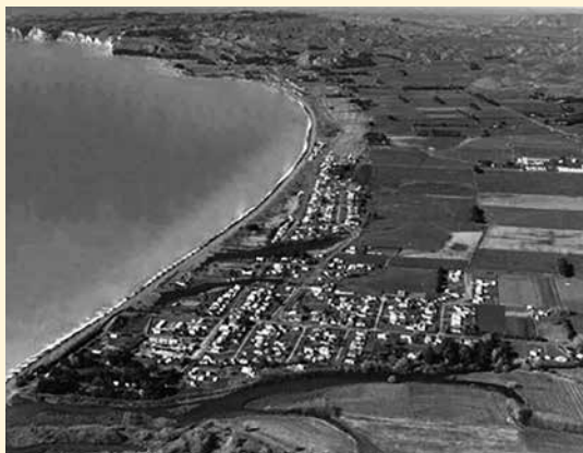
Aerial view of the Haumoana area.
