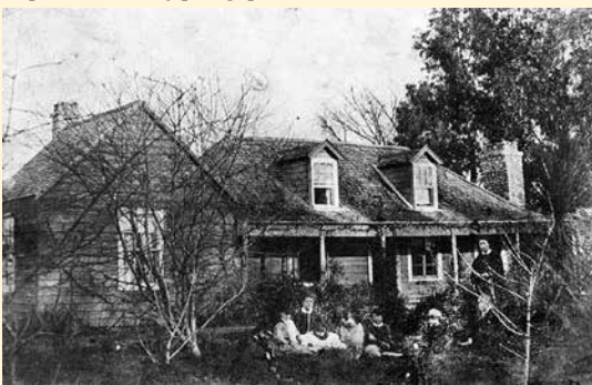
The first Clive Grange was built by Joseph Rhodes. Photo shows his family seated in front of the building.
