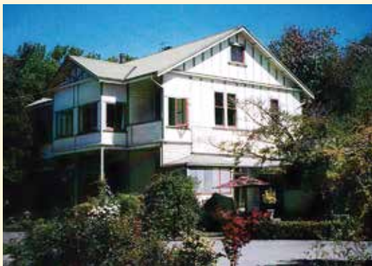
The homestead before it was destroyed by fire in 2009
