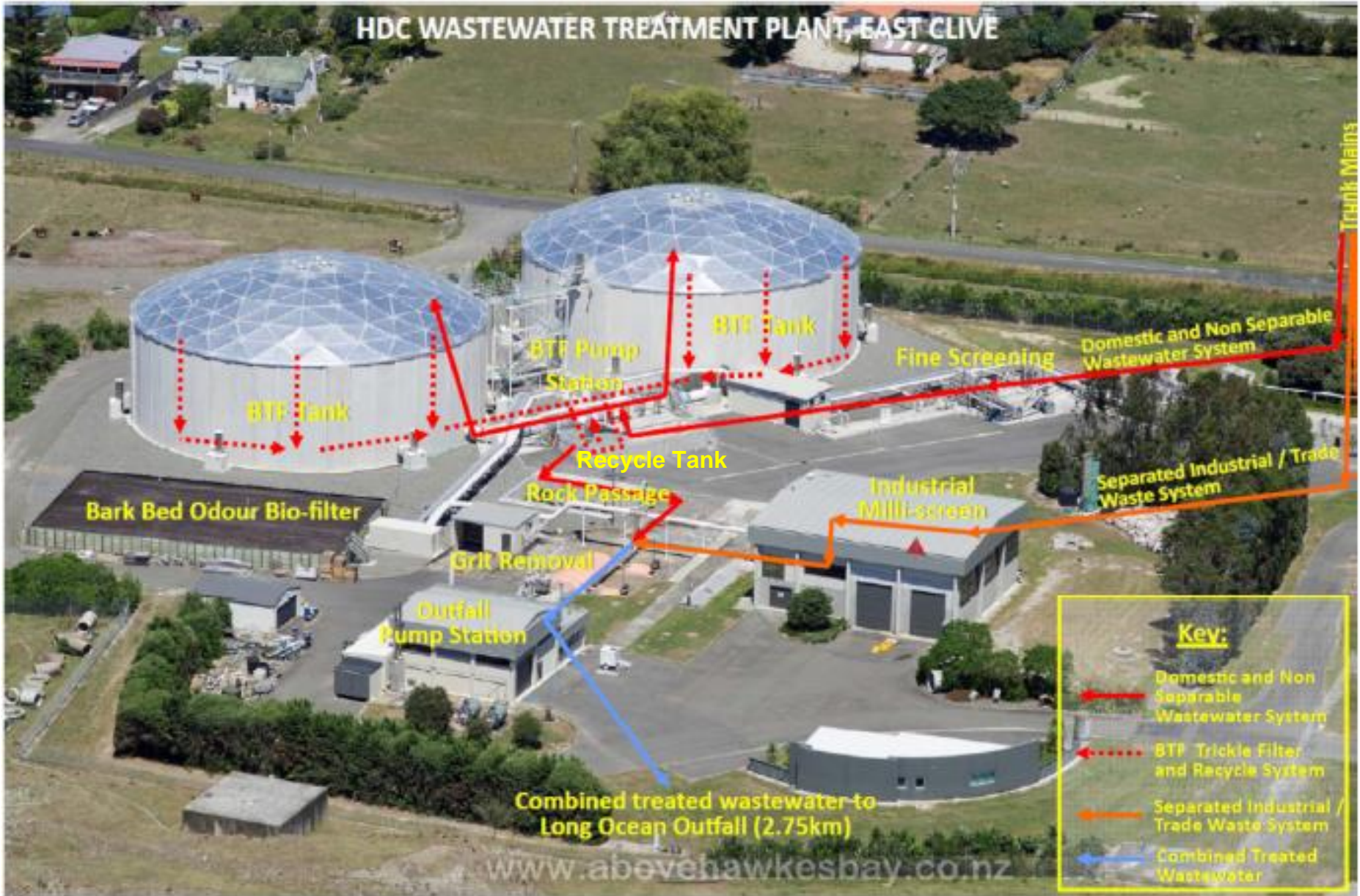
Figure 1: HDC Wastewater Treatment and Flow Paths
