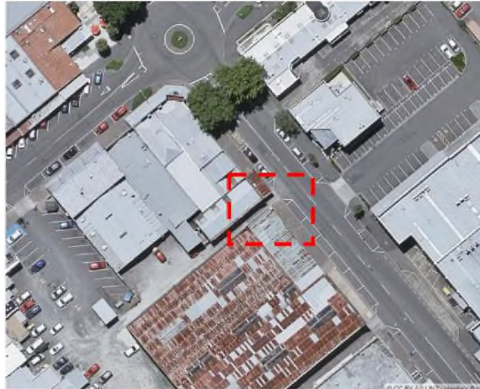
Figure 3: Existing vehicle access point
