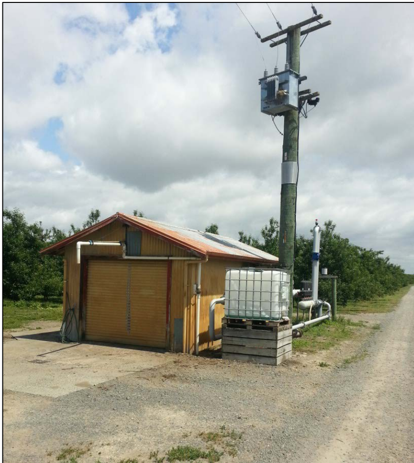
FIGURE 7: CHEMICAL STORAGE AND PUMP/BORE AREA – 280 STATE HIGHWAY 2 NORTH
