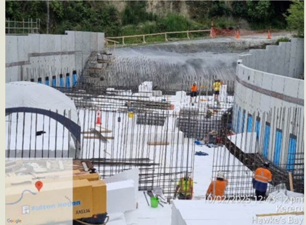
EPS installation in progress in the three cells.
