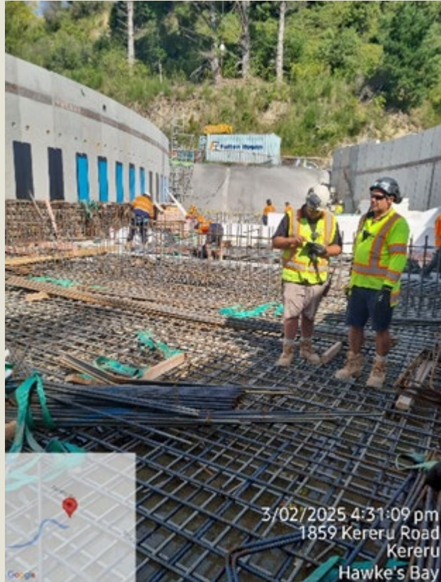
Upper headwall reinforcing steel installation.
