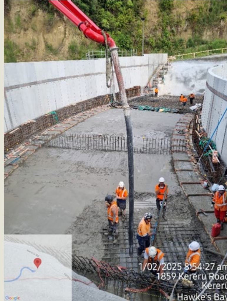
Concrete cast to base slab to lock in walls.
